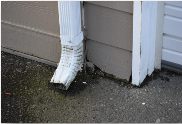
Downspouts in several locations are not channeling water away from building as needed
