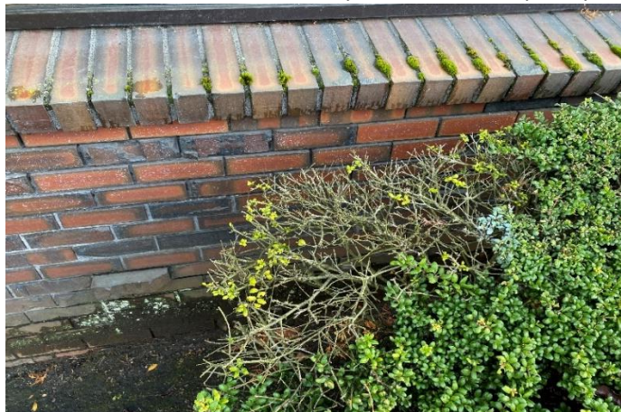
Brick base and soil/vegetation against masonry
