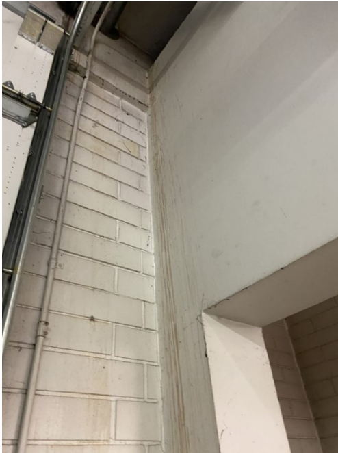
Signs of Water Intrusion – Engine Bay
