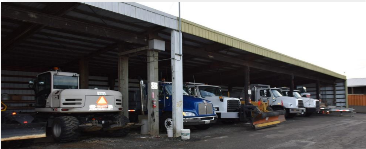
The “Lean to” provides covered shelter for Trucks and Street Equipment. The building isn’t deep enough to fit the longer trucks/equipment. Extending, adding roll-up doors, and enclosing the space with good ventilation will help to preserve expensive mobile equipment assets.
