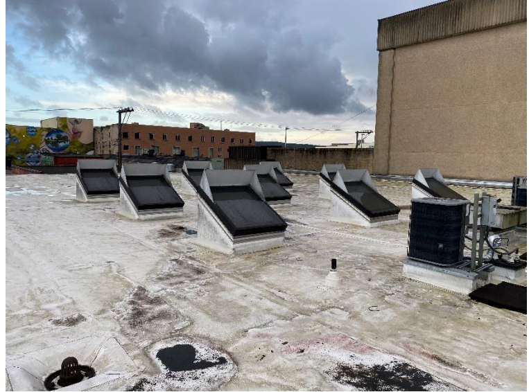
Library roofing membrane, skylights, some ponding water, mud on roof
