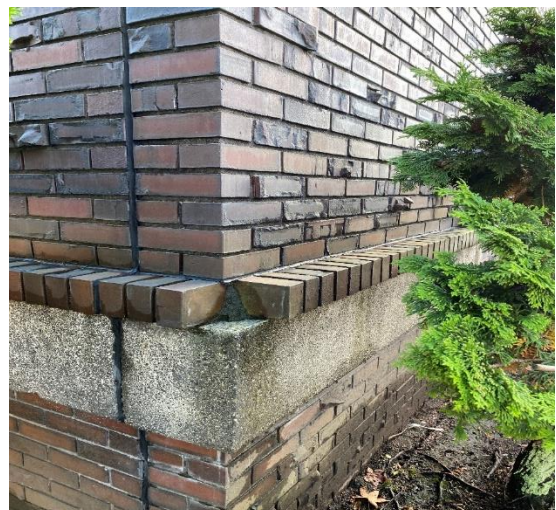
Brick veneer expansion joint. Missing broken brick ledge
