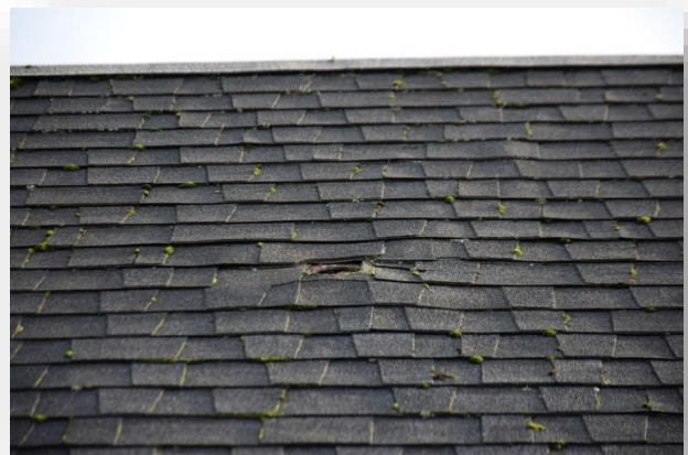
Roofing of Barn Building needs patching and eventual reroof. The Barn is structurally sound overall
