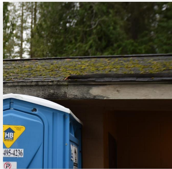
Sam Benn Park – Roofing in bad shape
