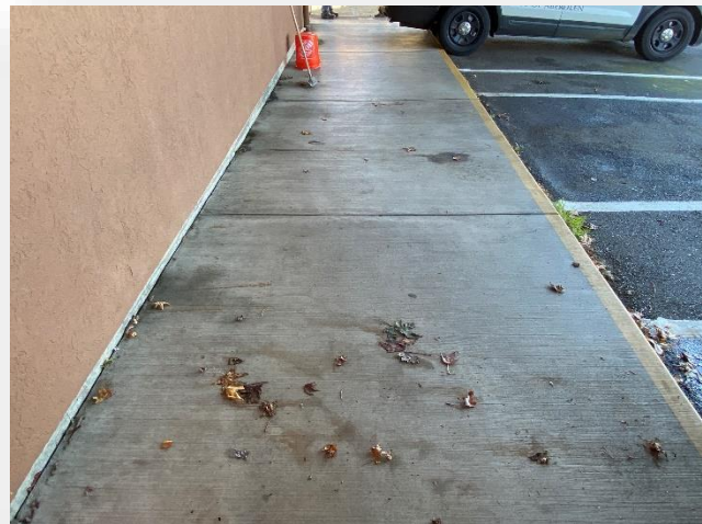
Police Headquarters – Site is settling away from structure
