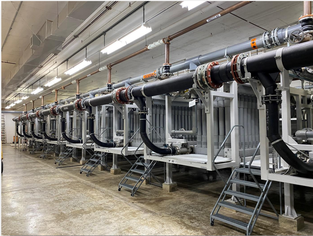
The filtration system. The 8-membrane microfiltration modules remove 99.9% of particles.
