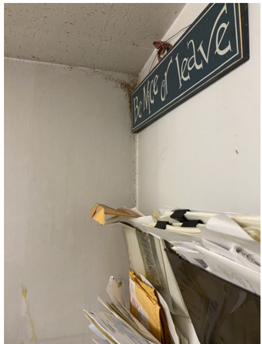
2 nd Floor Office – Signs of Mold
