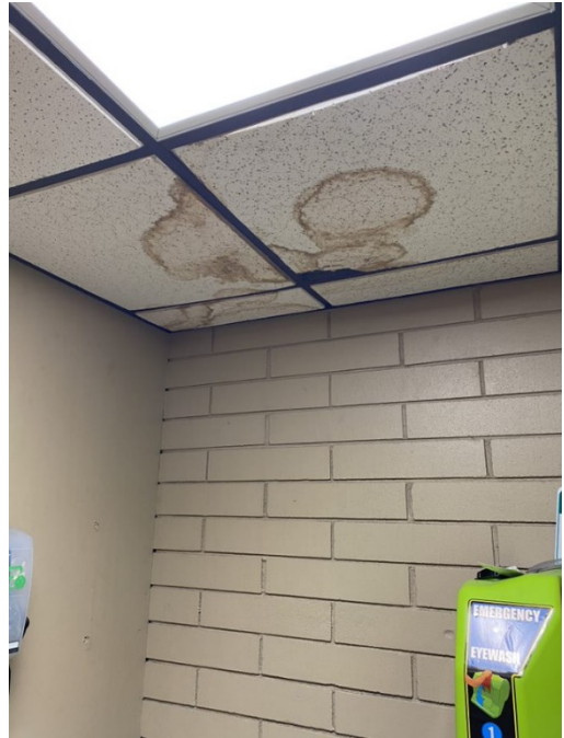
Typical Ceiling Tile Damage from Water
