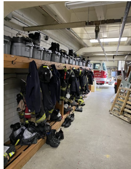
FIRST FLOOR PPE AREA SHARES VEHICLE BAY AREAS AND SAME HVAC SYSTEM
