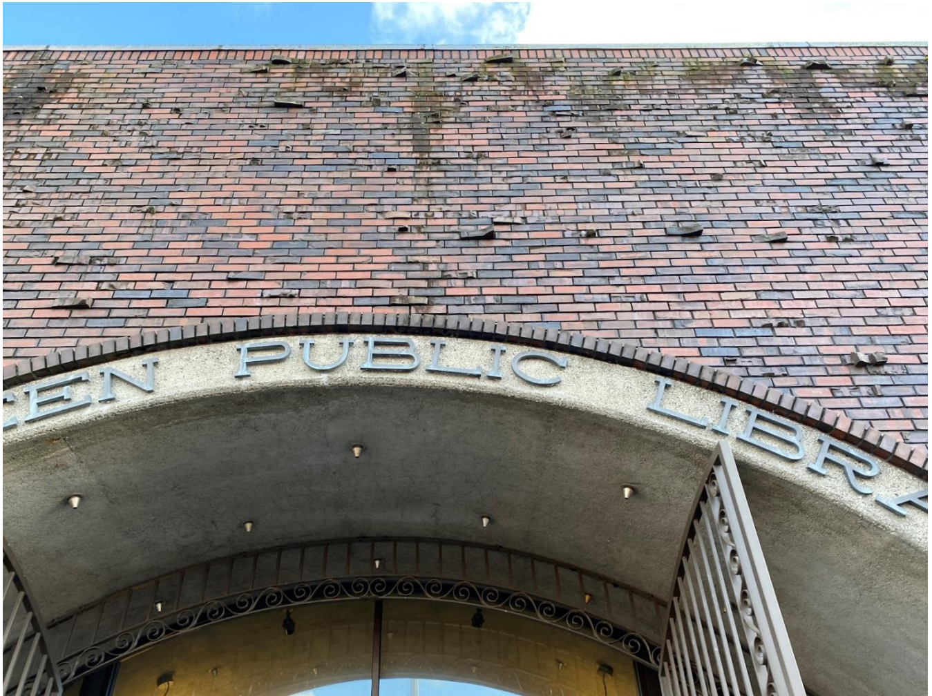
Aberdeen Public Library Entry and damaged brick facade
