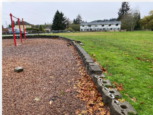
North Abedeen Playfield – Split-face CMU blocks separating play area from playfield have come loose and need to be resecured.
