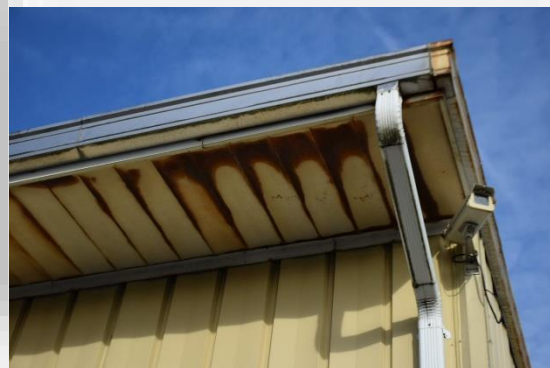
Each building exterior is showing signs of age. The metal siding shows signs of water intrusion in several locations on each building.
